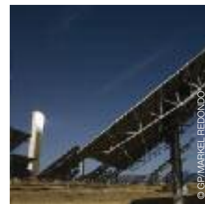
image The PS10 Concentrating Solar Tower Plant in Sevilla, Spain.
