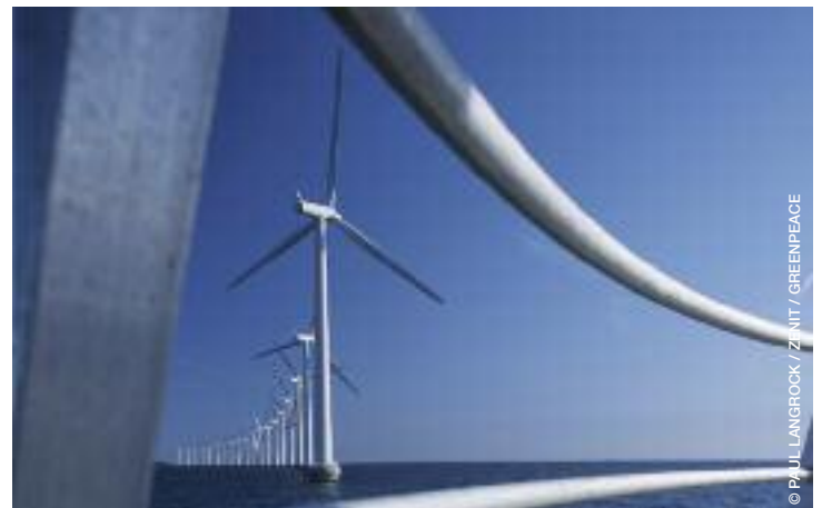
image Off shore windfarm, Middelgrunden, Copenhagen, Denmark.
