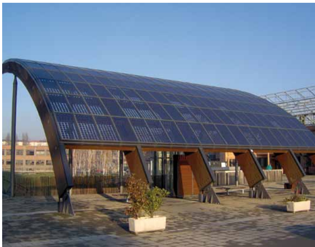
Totem fotovoltaico, Environmental Park (TO)
